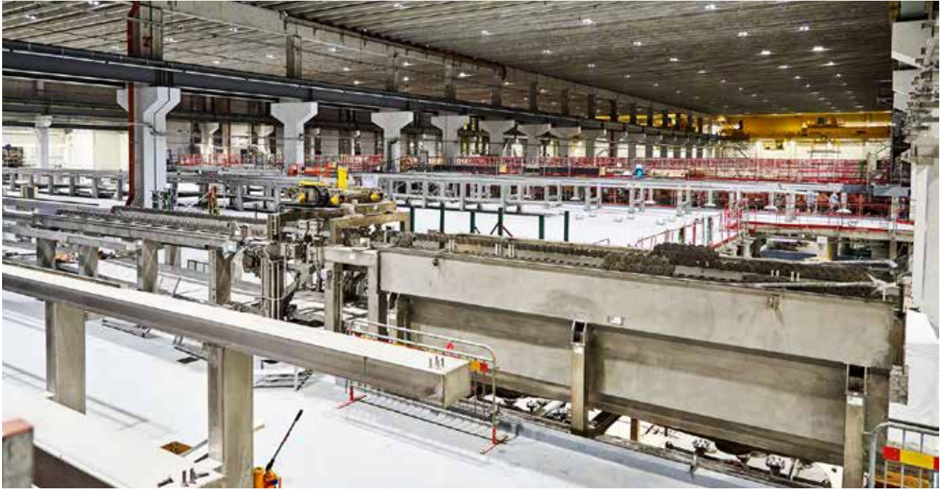
The tankhouse machine area during ongoing construction in March 2026
