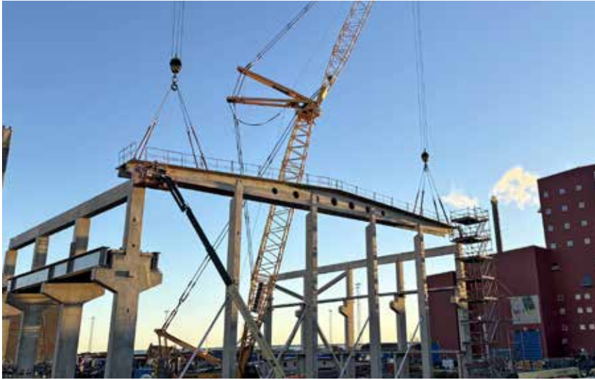
Roof truss prepared with integrated sprinkler systems, installed at ground level before being lifted into place
